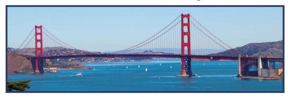
Once the longest suspension bridge in the world, the Golden Gate Bridge in San Francisco Bay is perhaps the most photographed bridge by far. A suspension bridge is one that has several tower structures with cables connecting them and giving the roadway support. Completed in 1937, it took four years to build.
