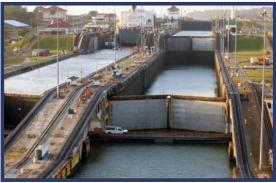
Begun in 1881, the work on the Panama Canal took over 30 years to finish. Since 1914, it has provided a waterway for ships passing through the narrow land area between the Gulf of Mexico and the Caribbean Sea. This 48-mile passage has locks at each end to raise ships up above sea level. A lock for ships is like a water elevator that can raise or lower them. The canal is considered by some to be one of the seven wonders of the modern world.
