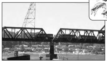
While the addition of trusses increases the strength of a beam, truss bridges also have limits on their maximum practical length.
