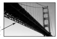
Fig. 49 - The use of trusses on the road decking of a suspension bridge.
