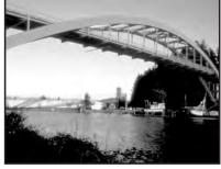
Not all arches are made from stone. Modern arches are made from steel frames.
