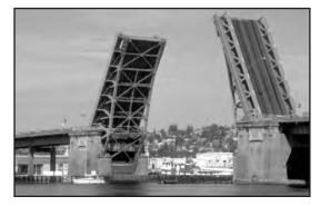
Fig. 52 Bascule Bridge opening for shipping.
