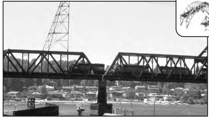
While the addition of trusses increases the strength of a beam, truss bridges also have limits on their maximum practical length.
