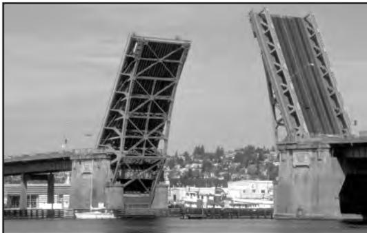
**Fig. 52 Bascule Bridge opening for shipping.**
