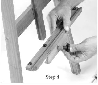
**Step Four - Assemble the Painting Trays:** Locate 2 metal guides (H & I), 2 black knobs (K), 2 black washers (J) and 2 metal washers (L).
