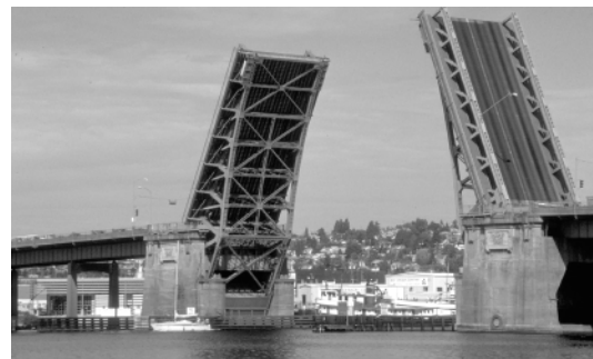
A bascule bridge opening for shipping
